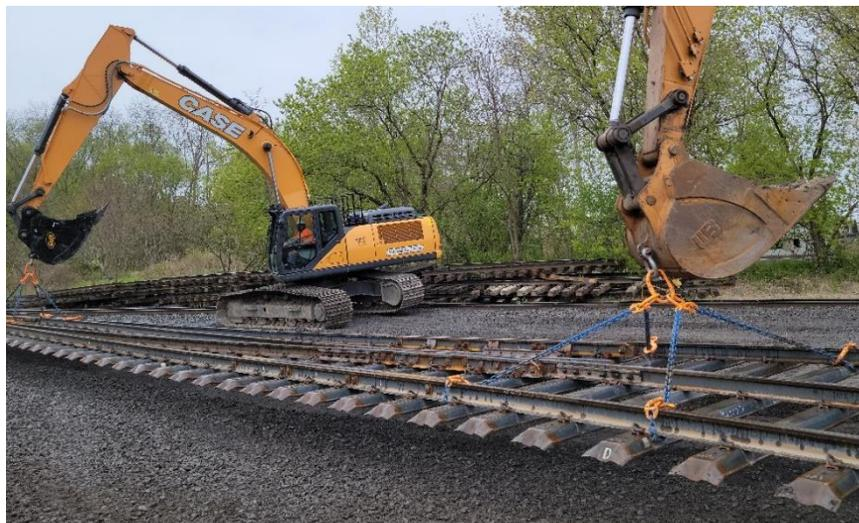
“The steel tie is resistant to damage, corrosion and deterioration. It’s 100% recyclable making it the superior option for usage in a busy rail yard such as Geneva,” states Joann Armstrong-Bruch, General Manager of Finger Lakes Railway.
